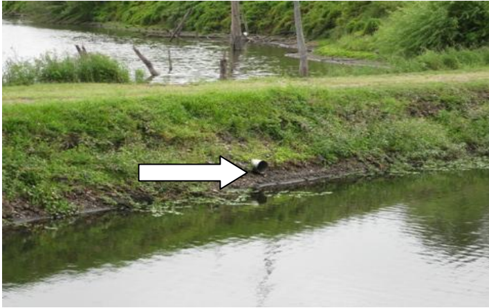
Arrow indicates transfer pipe
