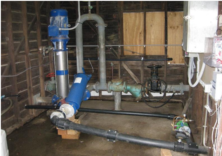
Existing Pumping Station
